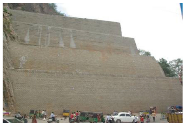
Fig. 29 Overall view of 41 m high wall
