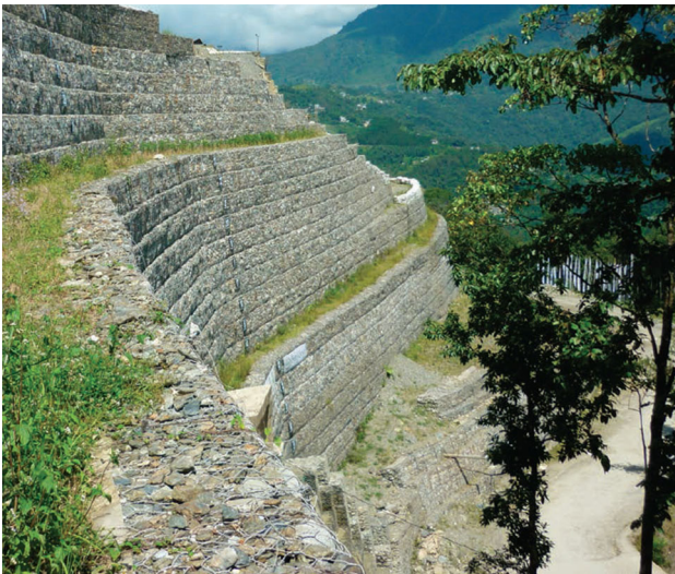
Fig. 33 Stone filled gabions as facing elements [36]
