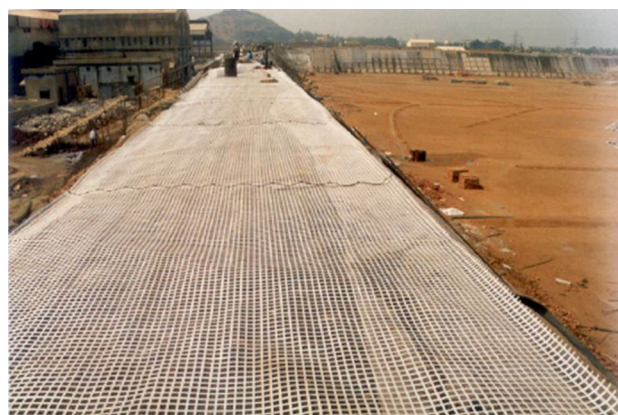
Fig. 44 Geogrid reinforcement in landfill embankment
