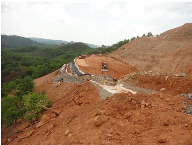
Fig. 35 Tiered embankment during construction
