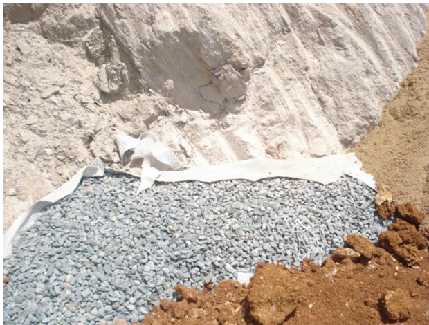
Fig. 22 Close up view of chimney drain and the geotextile filter
