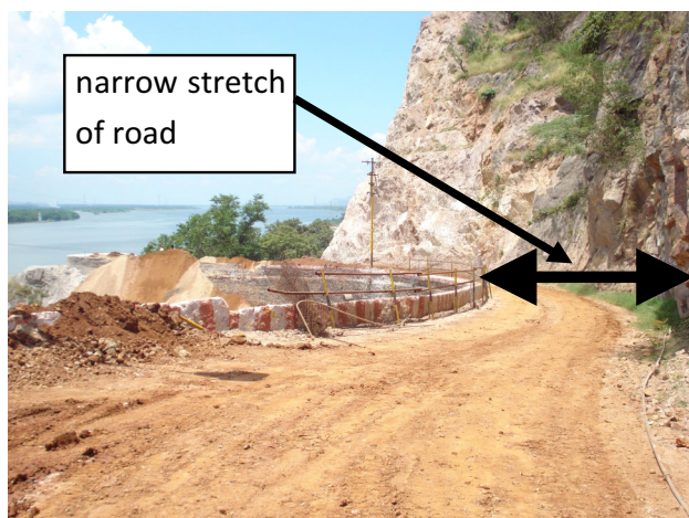
Fig. 18 Typical narrow section of ghat road at Vijayawada
