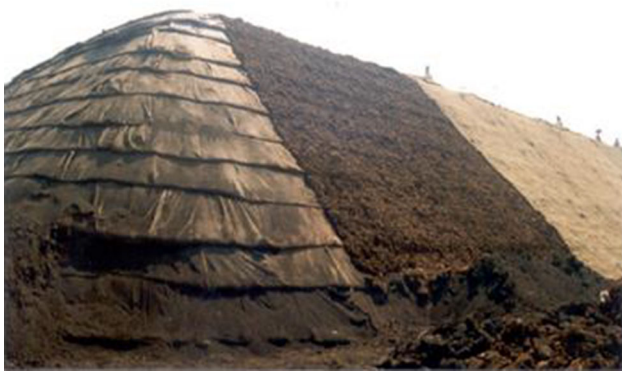
Fig. 45 Wrap around facing of slope surface covered with coir mat
