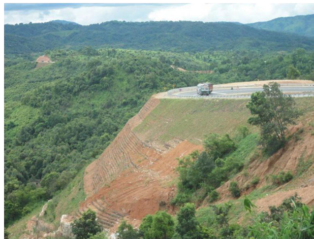
Fig. 37 Completed slope with road traffic and surface vegetation
