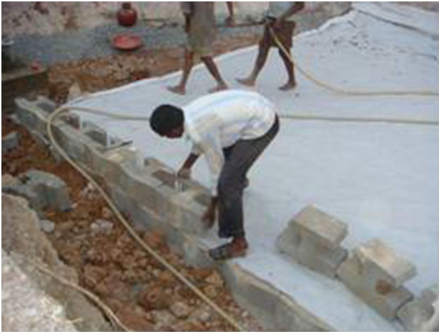
Fig. 25 Laying of the blocks
