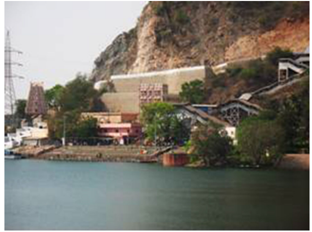
Fig. 28 22.5 m high wall
