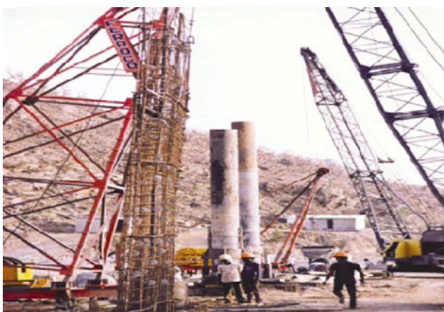
Fig. 34 Jacking of stop end pipes
