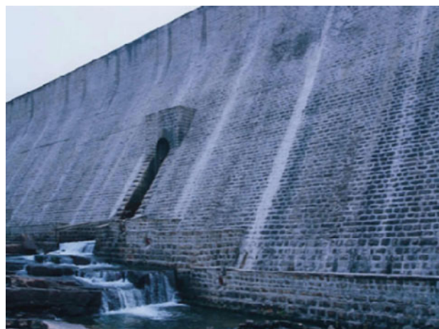
Fig. 49 Sluice of Pagara dam
