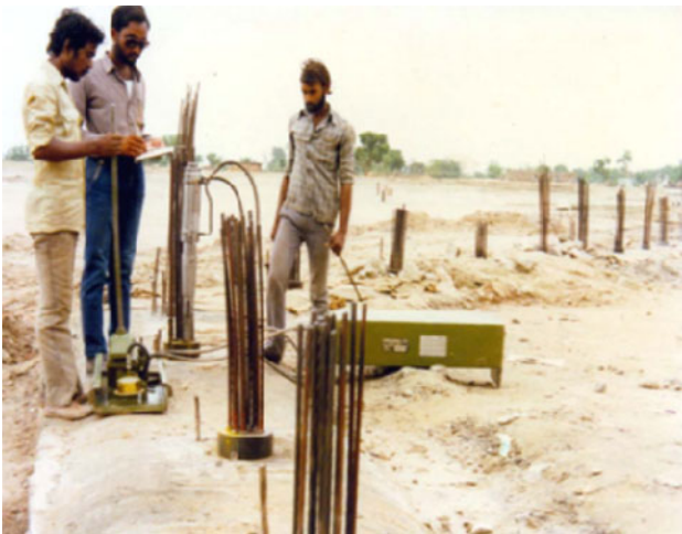
Fig. 39 Post tensioning of anchors
