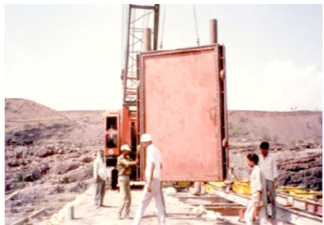
Fig. 15 Lowering of sluice gate
