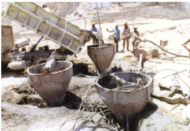
Fig. 33 Pouring of concrete in diaphragm wall panel
