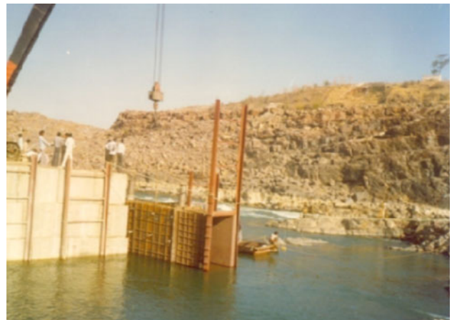
Fig. 14 Fixing of construction sluice
