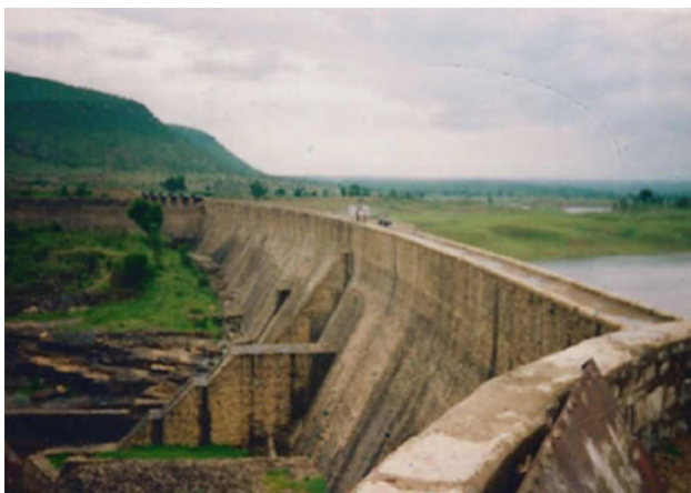
Fig. 51 After grouting treatment (Pagara dam)
