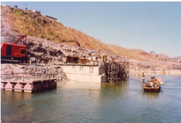
Fig. 10 Launching of blocks
