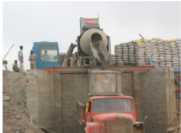
Fig. 31 Preparation of concrete
