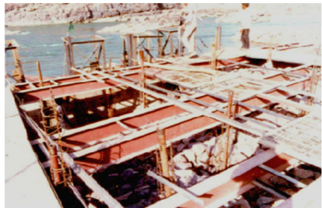
Fig. 11 Preparation for colgrouting
