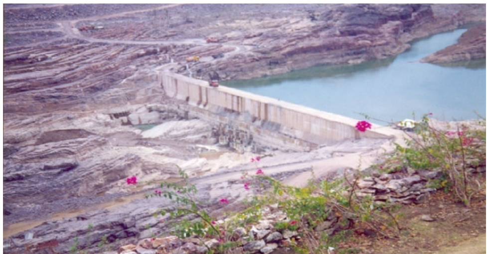
Fig. 17 Completed upstream coffer dam
