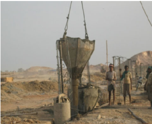
Fig. 30 Lowering of tremie pipes
