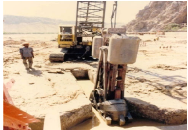
Fig. 28 Trenching and chiselling of panels
