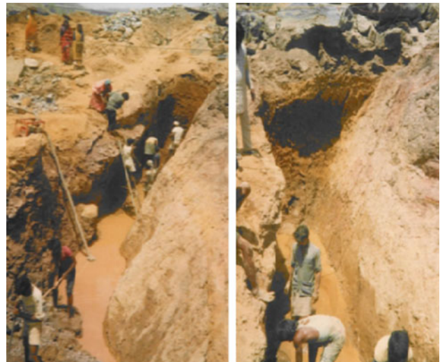
Fig. 7 Shear seams in foundation
