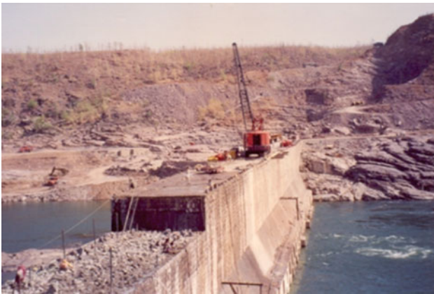
Fig. 16 Masonry work over RCC blocks
