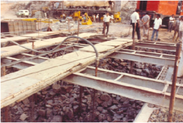
Fig. 12 Preparation for colgrouting
