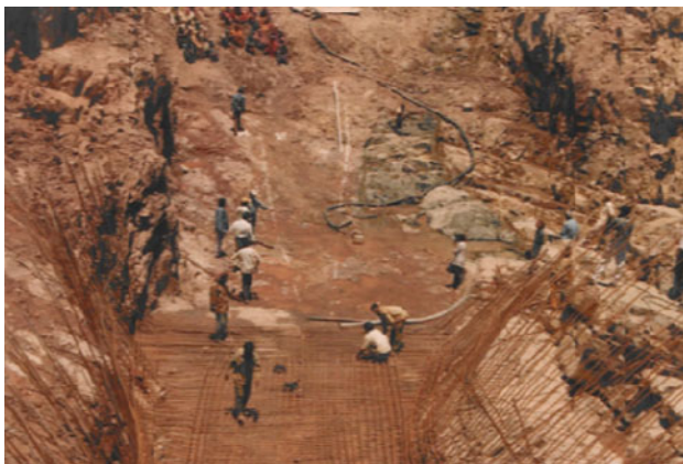
Fig. 4 Treatment of fault zone
