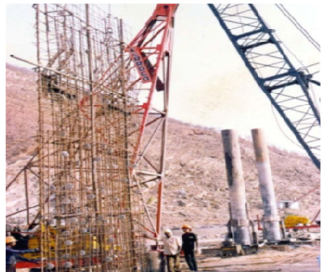
Fig. 29 Lowering of reinforcement in panel
