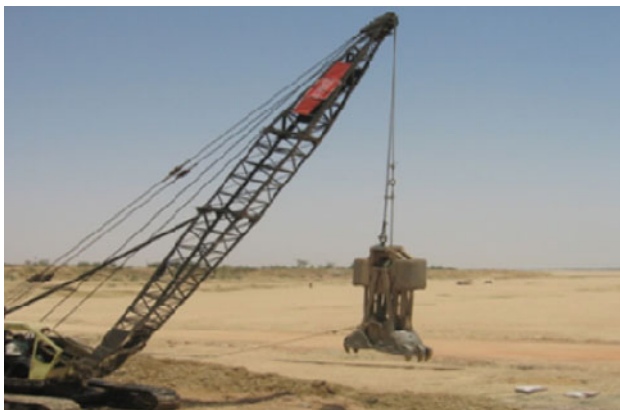
Fig. 27 Trenching and chiselling of panels
