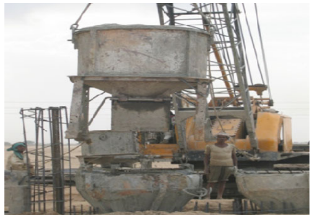
Fig. 32 Pouring of concrete in diaphragm wall panel
