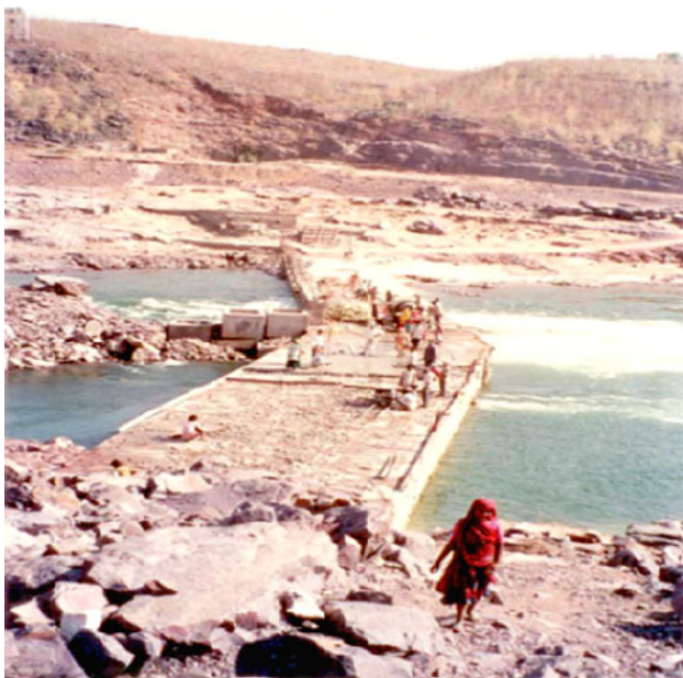
Fig. 18 Completed downstream coffer dam
