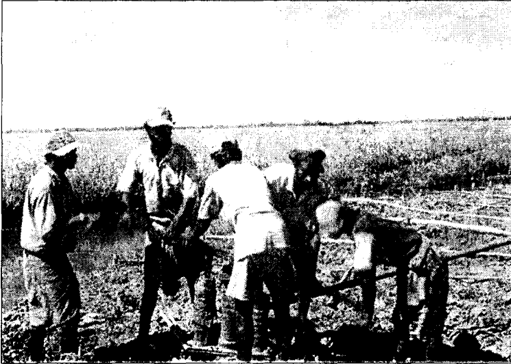
FIGURE 4 : Auger Boring with Hand Operated Mud Pump
