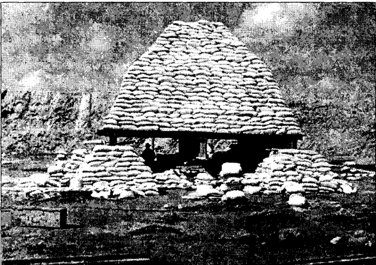
FIGURE 7 : Improper Design of Loading Arrangement
