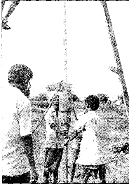
FIGURE 2 : Crude Method, No Safety Measures, No Assurance of Vertical Application of Load
