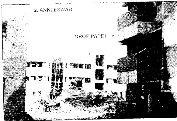
FIGURE 43 : After Collapse of Structure
