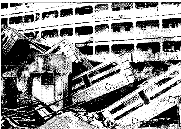
FIGURE 37 : Collapsed Building in Surat
