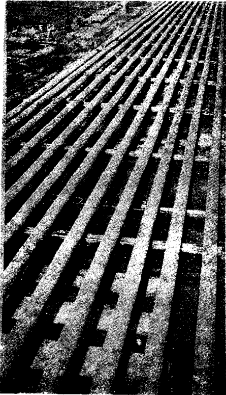
FIGURE 91 Strings of Pipe kept ready for Pulling
