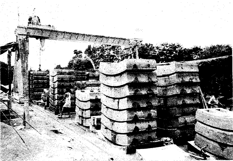
FIGURE 37 Stacks of Liner Segments ready for Placement
