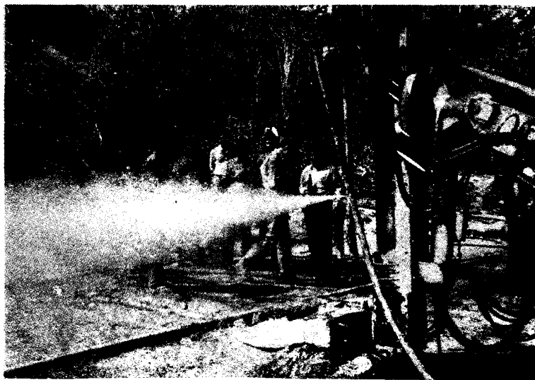
FIGURE 14 Jetting Action of C-6 Ring on Ground at Ch. 151
