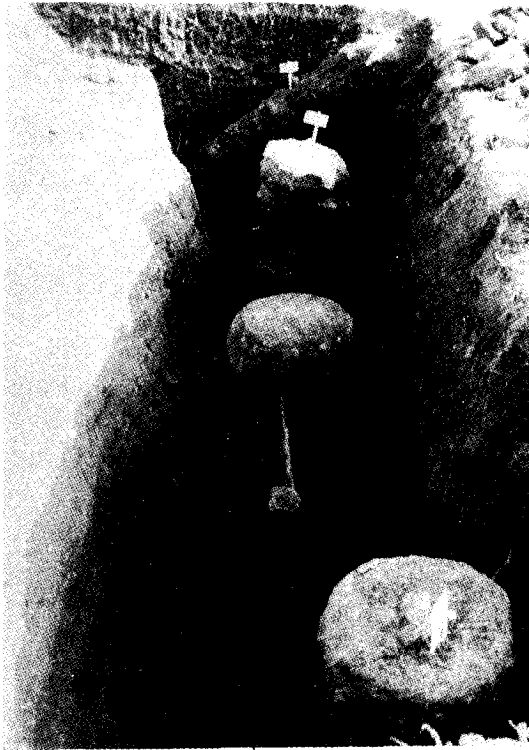
FIGURE 10 Close up view of Jet Grout Columns formed in Trial Study
