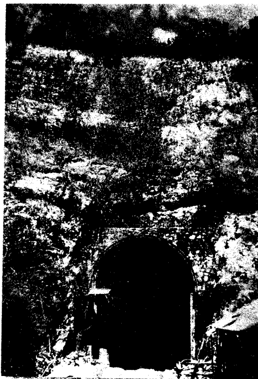
FIGURE 15 A View of Lelligumma Tunnel at Koraput Face
