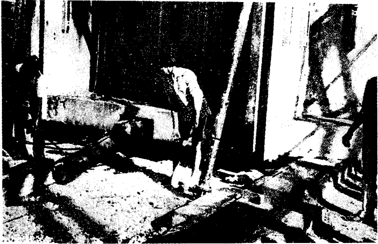
FIGURE 79 Shifting of Crib Unit with Hydraulic Jacks
