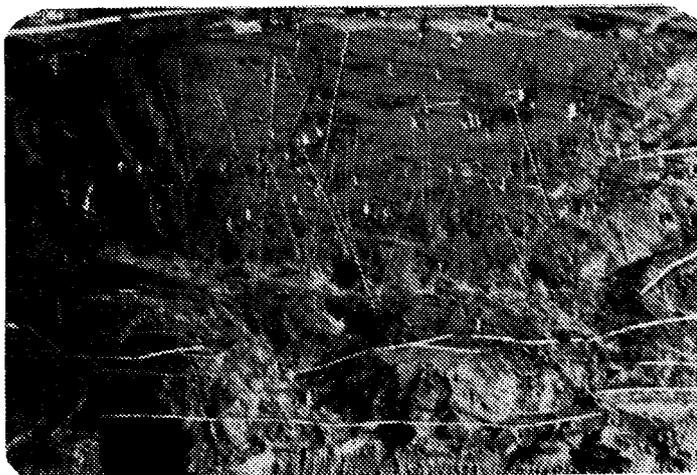
FIG 58. INSTALLATION OF GRANULAR PILES AT THE BASE OF THE RCC RAFT
