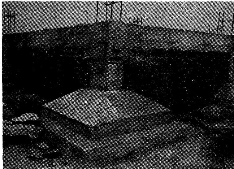
**FIG 21. PLINTH BEAM AFTER REMOVAL OF SIDE SHUTTERING**
