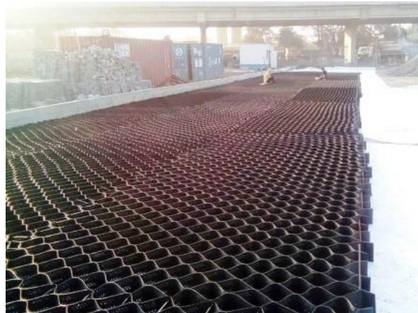
Fig. CY-4(b): First layer of geocells laid over nonwoven
