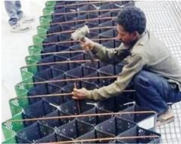
Fig. FS-9: Laying of geogrids and geocells
