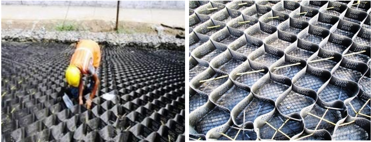
Fig. LF-19: Tying StrataWeb® geocells to StrataGrid™ geogrids
