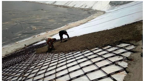
Fig. RE-4(b): Placing geocells in position
