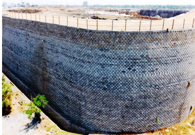
Fig. LF-8: The outer fascia of segmental precast concrete modular blocks
