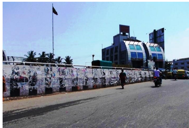
Fig. WL9: The completed wall
