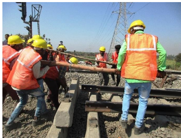
Fig. RW-7: Removal of sleepers
