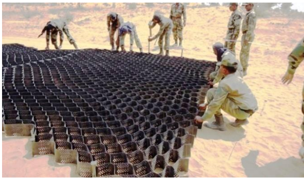
Fig. PV-5(a): Laying the geocell panel
