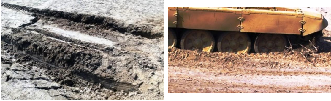
Fig. PV-6: Heavy tracked vehicle rutting deep into the unpaved subgrade; the pictures highlight depth of ruts
