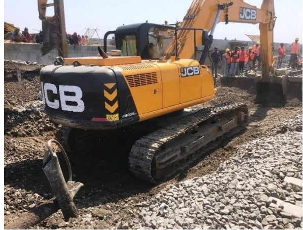
Fig. RW-9: Removal of sub-ballast / blanket material
