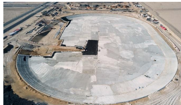
Fig. RE-2(b): Bed being concreted
