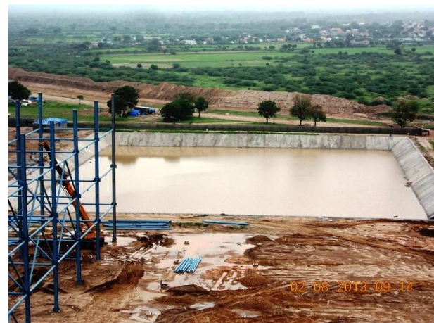
Fig. RE-5(d): The completed reservoir
