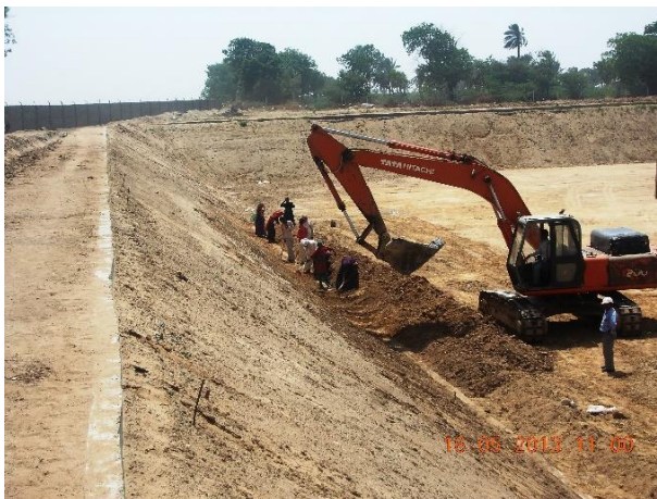
Fig. RE-5(c): Infilling with concrete
