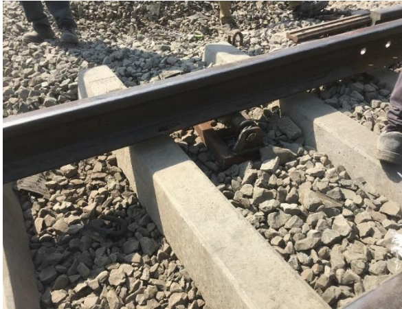
Fig. RW-23: Replacing rails on sleepers
