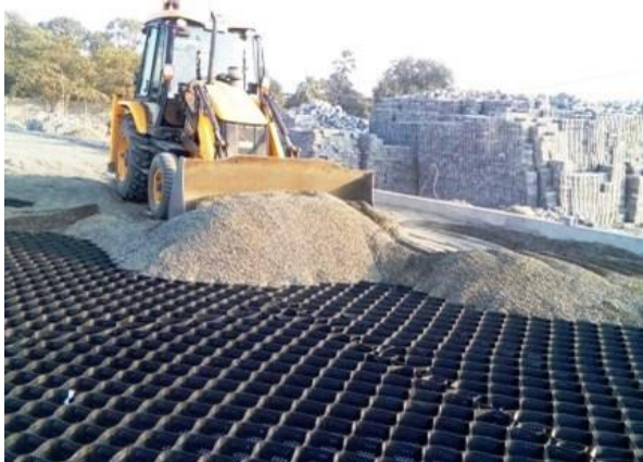
Fig. CY-4(c): Infilling of geocells
