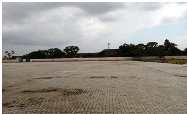
Fig. CY-5: Completed paving with geocells after one year
