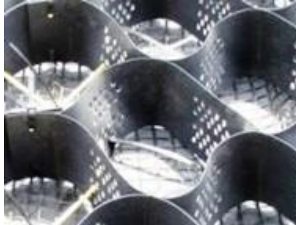
Fig. LF-24©: Geocells connected to geogrids with cable ties
