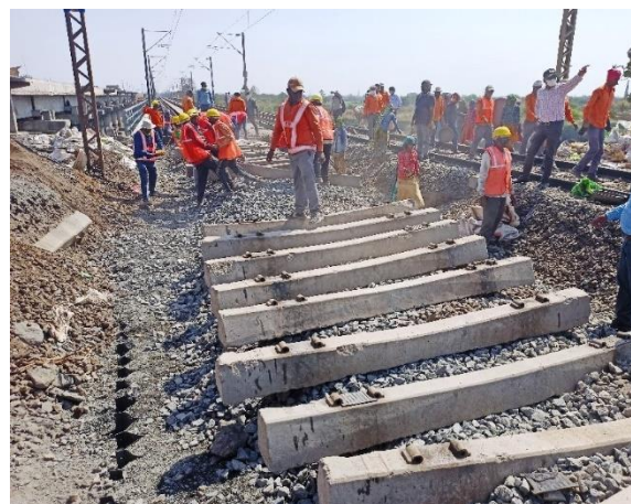
Fig. RW-22: Placing sleepers over ballast
