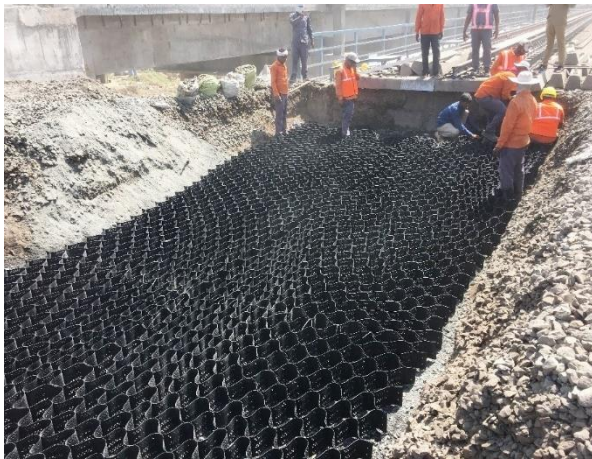
Fig. RW-16: Bottom-most geocell layer
