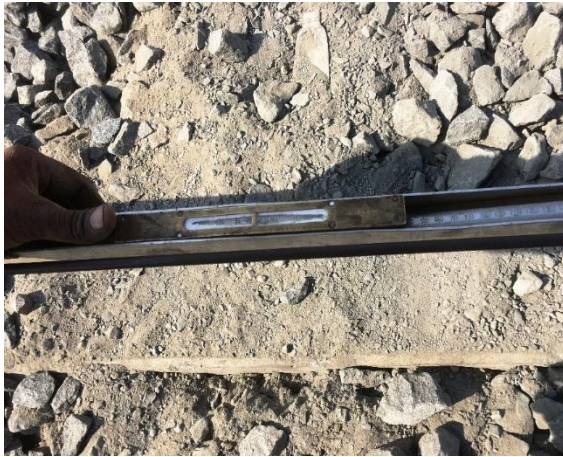
Fig. RW-27: Alignment check using Track gauge measurement device
