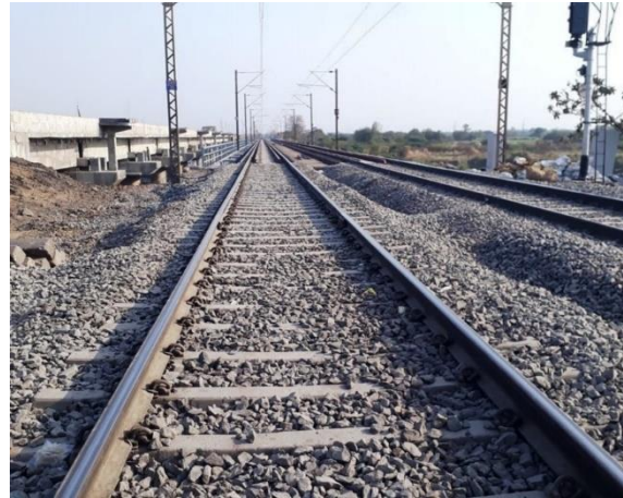
Fig. RW-28: Sides of sleeper packed with ballast
