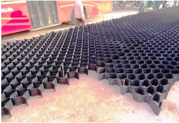
Fig. WL-6: The bottom-most geocell layer
