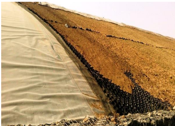
Fig LF-20(a): Geocells being infilled
