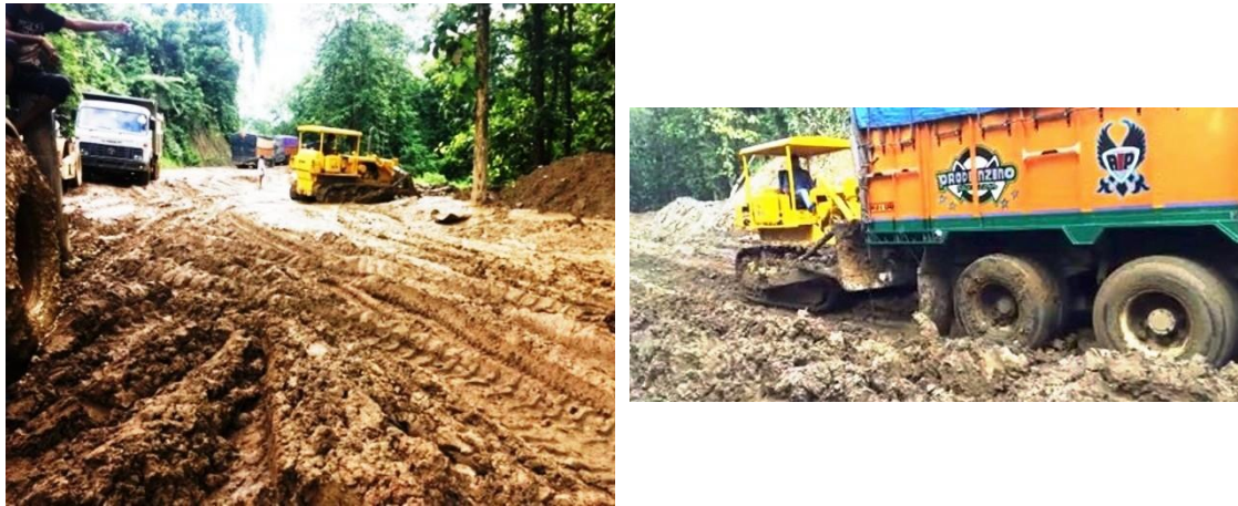
Fig. PV-8: NH-44 at Churaibari in July 2016 before rehabilitation
