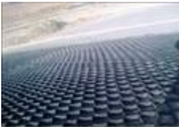
Fig. LF-25(a): Geocells laid out
