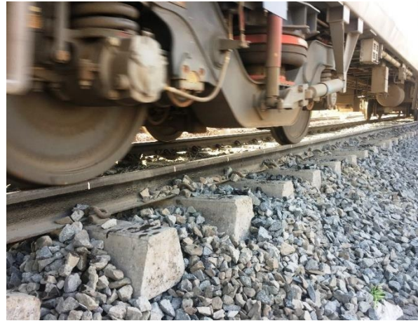
Fig. RW-31: Finished track surface at the bridge - approach transition zone
