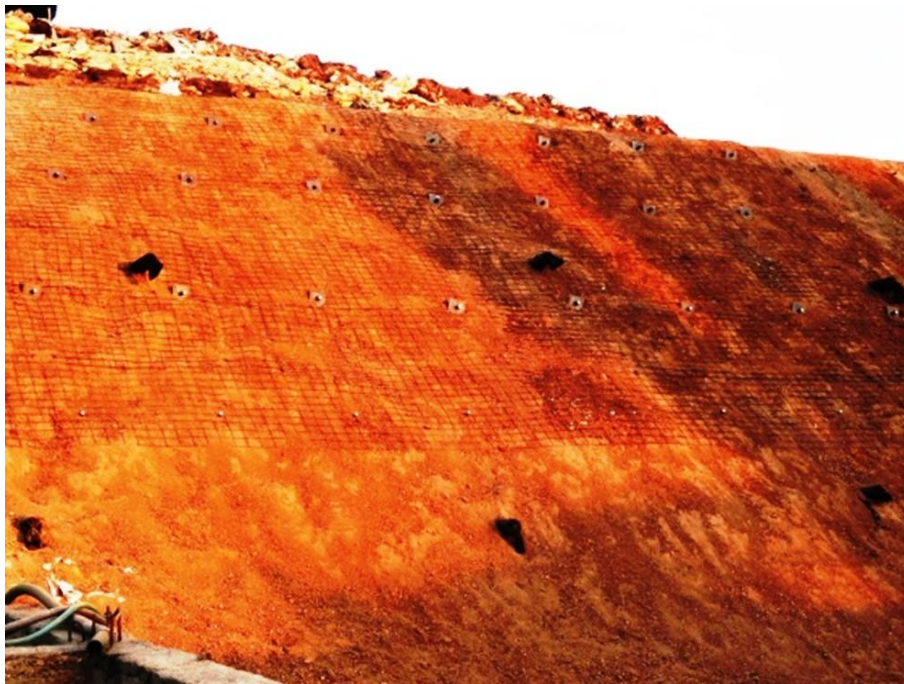
Fig. LF-14(b): West side: Soil nails for excavation in progress
