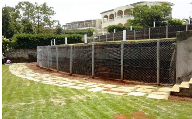
Fig. WL-4(d): Completed wall with mesh in front for green climbers
