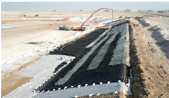
Fig. RE-2(a): Geocells on slope
