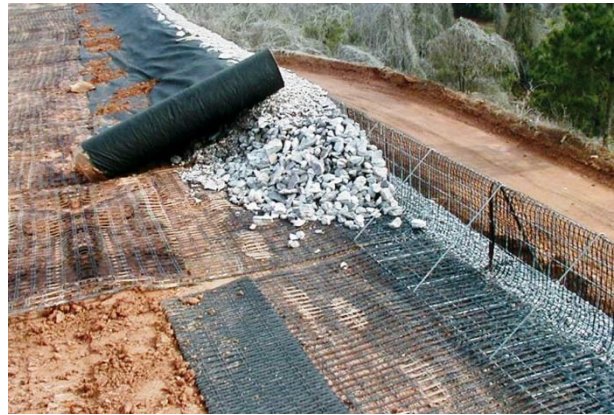
Fig. LF-2(b) Wire basket fascia in collapsed form
