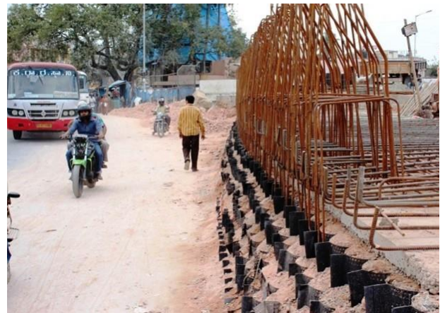
Fig. WL8: Friction slab (left) and crash barrier construction (right)
