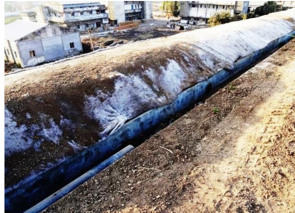
Fig. LF-17: Anchor mound at the crest holding the infilled geocells, the holding geogrid and the enabling tendon
