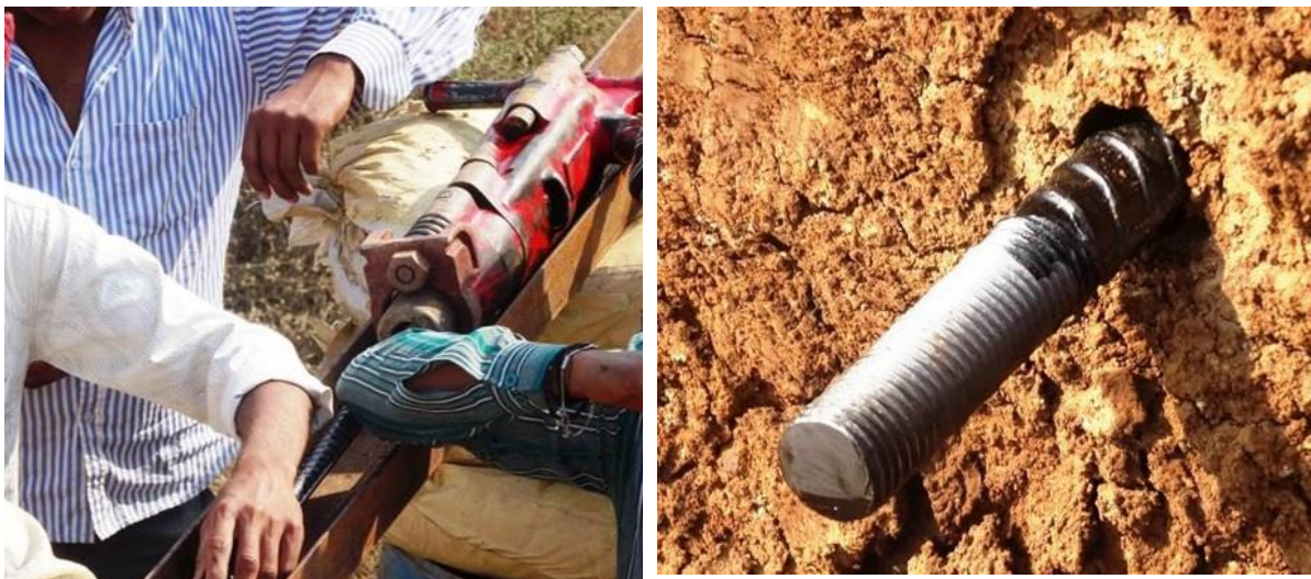
Fig. LF-16: Typical soil nail driving by specialist agency's team
