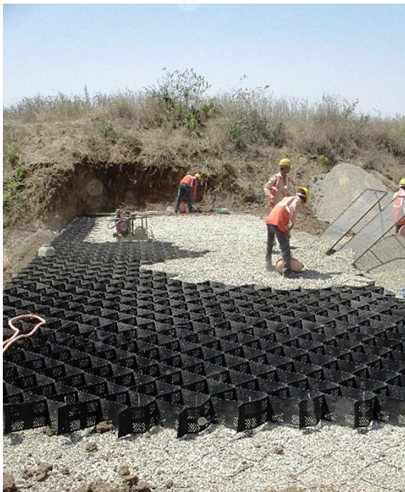
Fig. CD-5: Infilling of geocells with non-plastic soil
