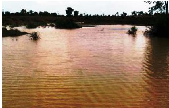
Fig. CD-8(b): Reservoir behind the check dam
