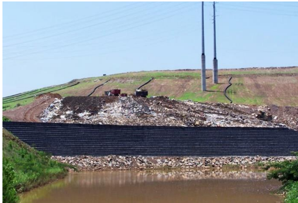
Fig. LF-2(a) The lower-level stone filled wire basket fascia
