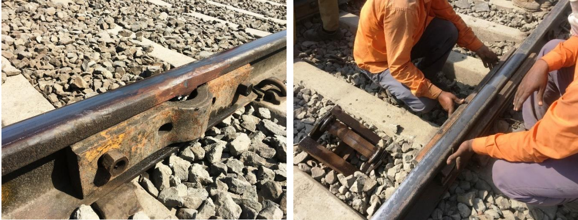
Fig. RW-25: Placing rail fish plates; left picture shows stiffening fishplate
