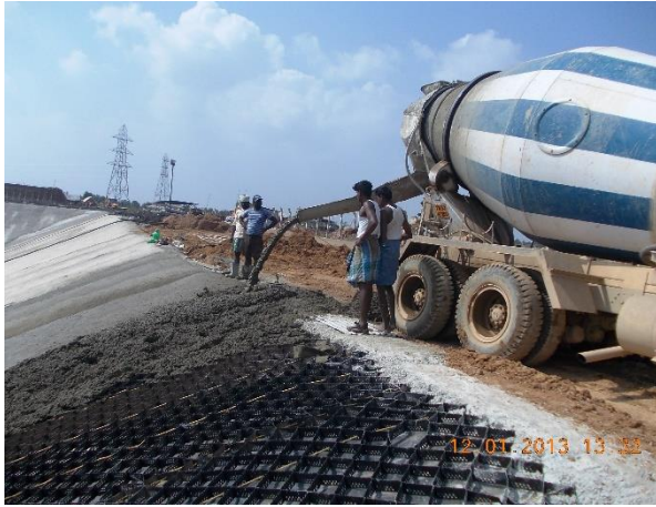
Fig. RE-3(c): Concrete infilling
