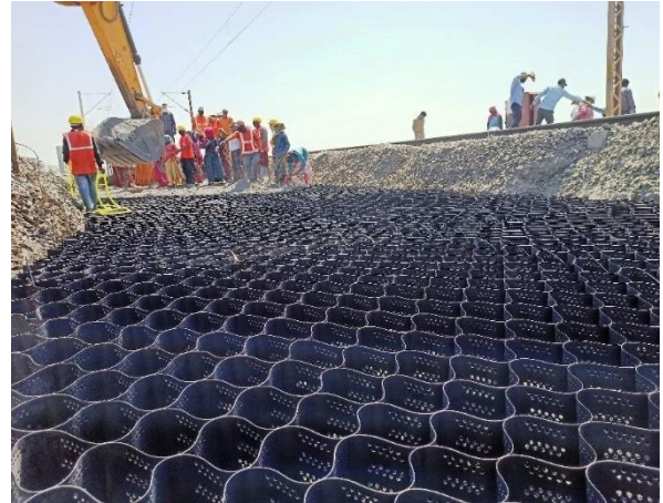
Fig. RW-20: Laying and infilling the topmost layer of geocells
