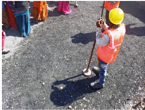
Fig. RW-12: Infilling of 100mm thick blanket layer
