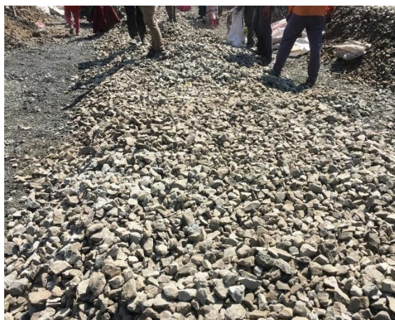
Fig. RW-21: Laying ballast over the blanket layer
