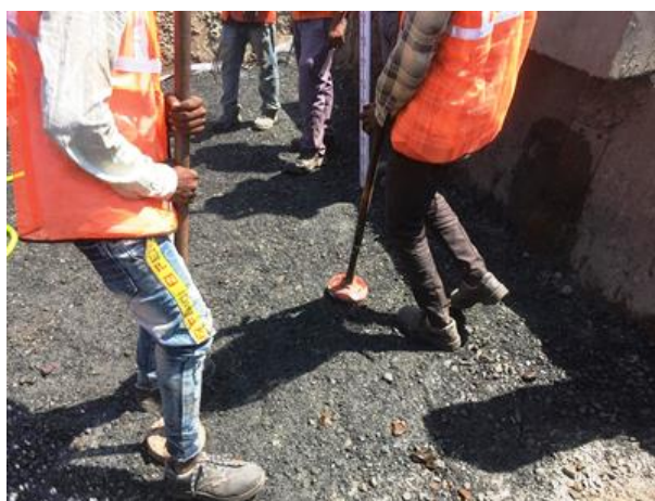
Fig. RW-18: Watering and compaction of bottom-most geocell layer
