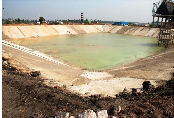
Fig. RE-3(d): The completed concrete lining
