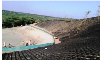
Fig. SC-11(b): Laying geocells
