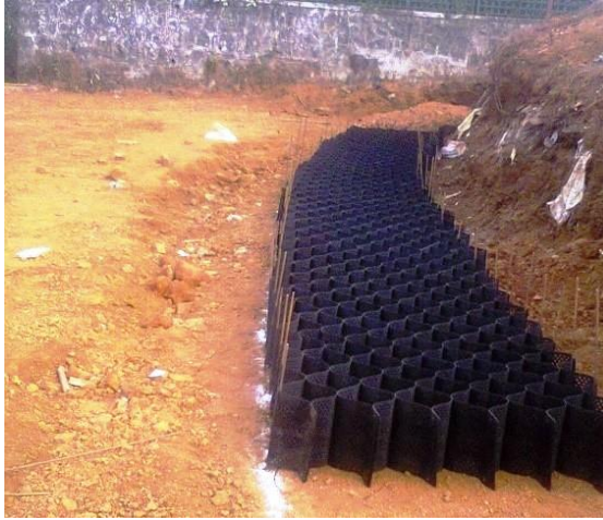
Fig.WL-4(a): Bottom-most row of geocells being laid out
