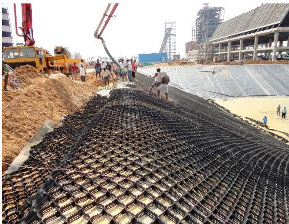
-Fig. RE-3(b): Geocells laid on slopes and anchored at the crests
