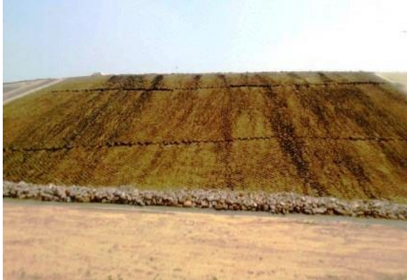
Fig. LF-26(a): Seeded infilling
