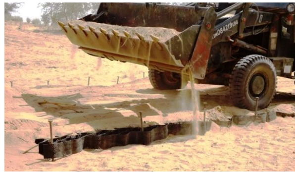
Fig. PV-5(b): Infilling geocell panels with local sand
