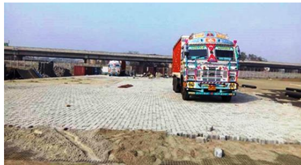
Fig. CY-4(d): Completed paving with geocells
