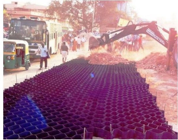
Fig. WL-7: Infilling the bottom-most layer
