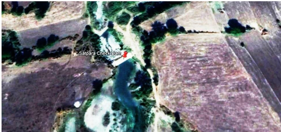
Fig CD-10: Satellite imagery of the Site after the construction of check dam (November 2018))
