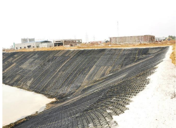
-Fig. RE-3(b): Geocells laid on slopes and anchored at the crests
