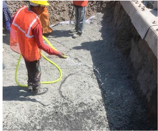
Fig. RW-13: Watering the blanket material for compaction
