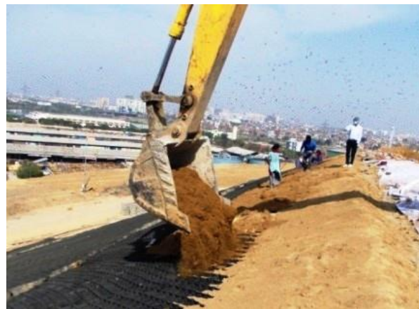
Fig. LF-25(b): Soil in-filling
