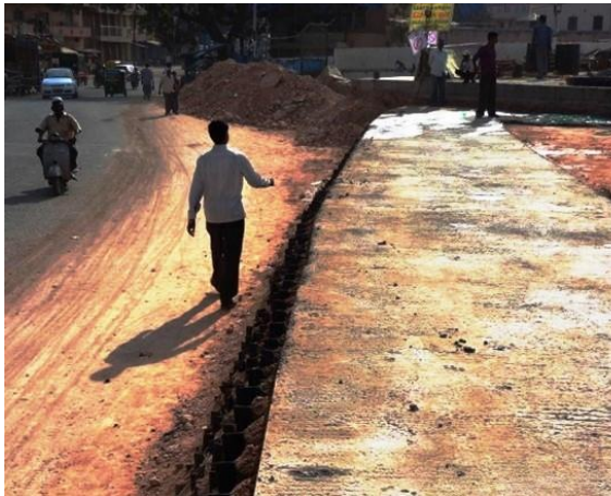
Fig. WL8: Friction slab (left) and crash barrier construction (right)
