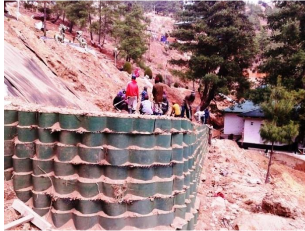
Fig. FS-11: Green façade of reinforced soil wall
