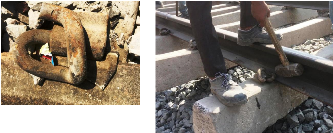
Fig. RW-26: Typical clip; Clamping between rail and concrete sleeper with rail clips
