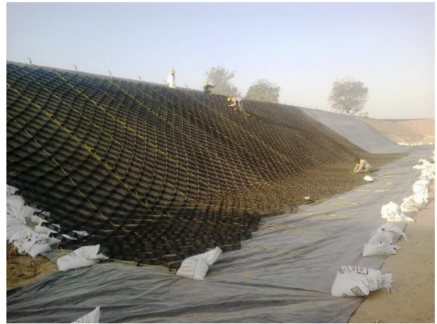
Fig. RE-5(b): Geocells laid on geomembranes overdressed slope
