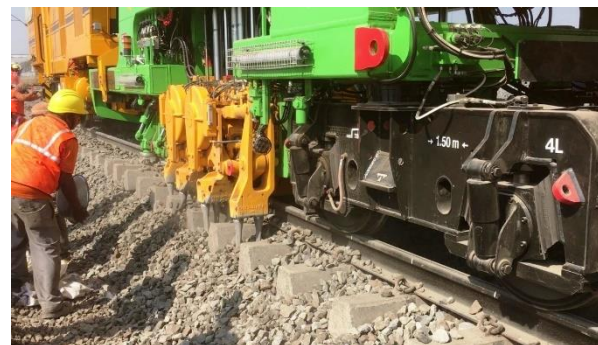
Fig. RW-29(b): Compaction of ballast by Dynamic Tamping Express machine
