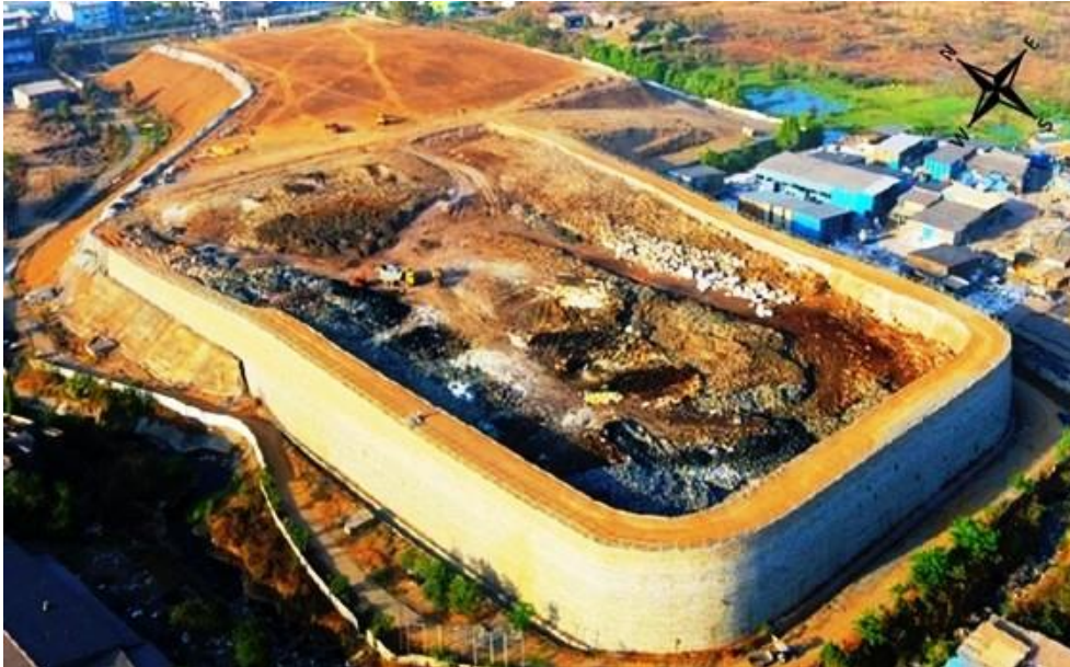
Fig LF-21: Bird's eye-view of the two types of containment structures; the conventional earth structure (above, North) and the reinforced soil structure (below, South); Note the differences in footprint areas
