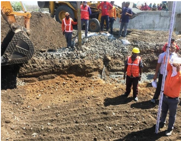
Fig. RW-10: Checking the excavation level
