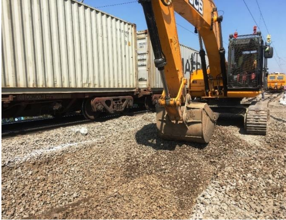
Fig. RW-8: Removal of ballast
