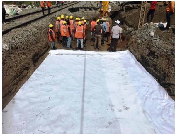
Fig. RW-11: Laying the nonwoven geotextile
