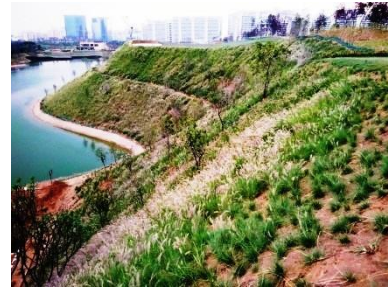
Fig. SL-11(e): Vegetated slopes by geocells
