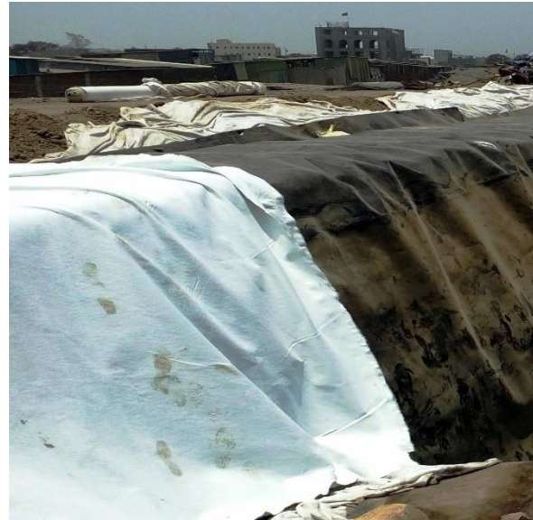
Fig. LF-7(b): Shroud of nonwoven-geomembrane-nonwoven sandwich laid over the inner slope
