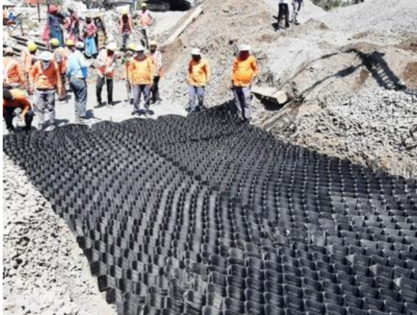
ig. RW-19: Laying and infilling of middle geocell layer
