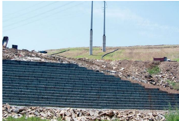
Fig. LF-2(d) Progressive construction of reinforced soil slope
