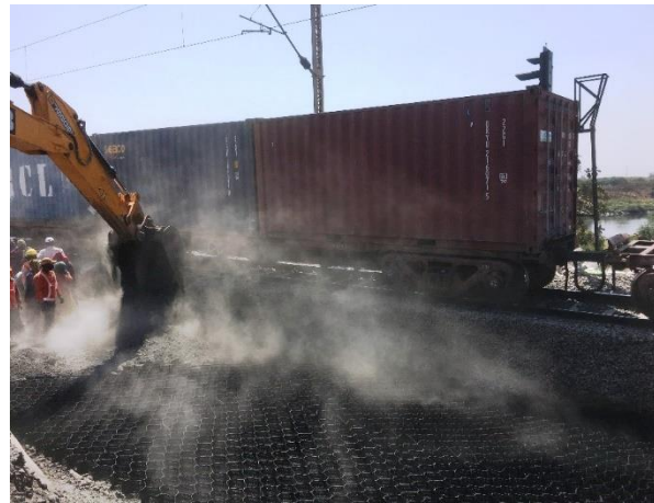
Fig. RW-17: Infilling geocells
