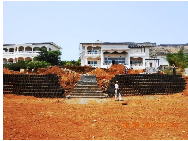
Fig. WL-4(b): Progressive construction of geocell wall
