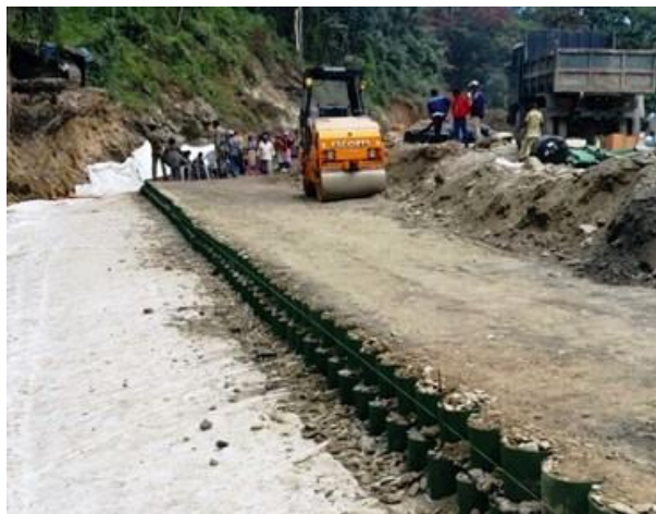
Fig. FS-10: Infilling and compaction for reinforced soil
