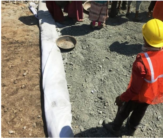
Fig. RW-12: Infilling of 100mm thick blanket layer
