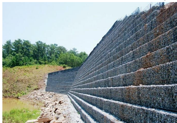
Fig. LF-2(e) Completed reinforced soil slope
