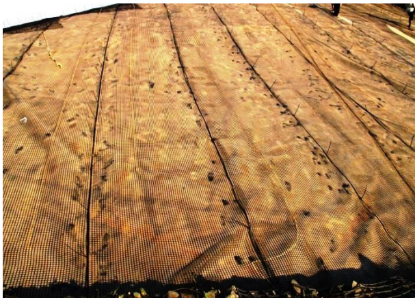
Fig. LF-18: StrataGrid™ Swi40 geogrid laid down the slope; adjacent widths secured together with cable ties
