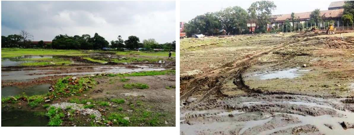
Fig. CY-2: Original Ground Condition (heterogeneous fill)
