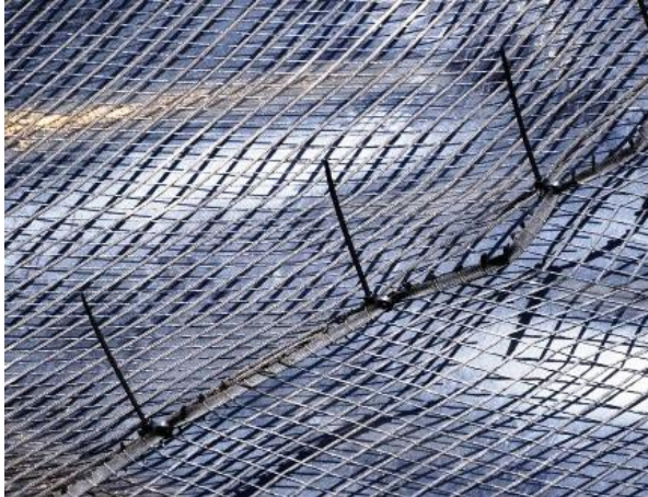
Fig. LF-25(b): Adjacent geogrids connected with cable tie
