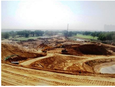
Fig. SC-11(a): Site grading
