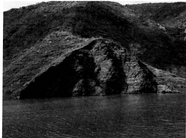
Plate 6 Failing Slopes in the Reservoir of Tehri Dam
