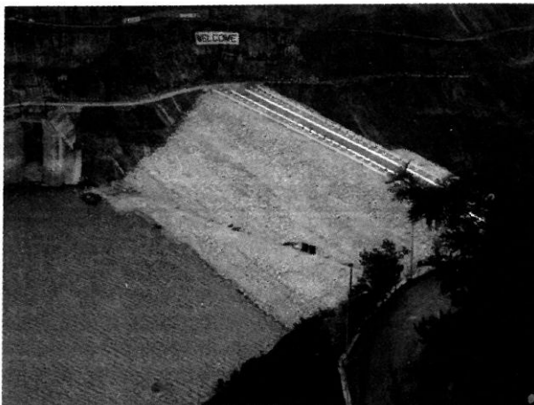
Plate 10 A View of the Earth and Rock Fill Embankment at Tehri Project
