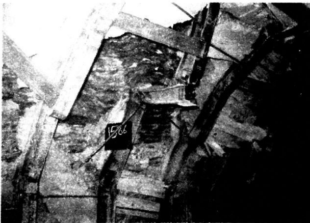
Plate 14 Another View of Tunnel through Squeezing Grounds
