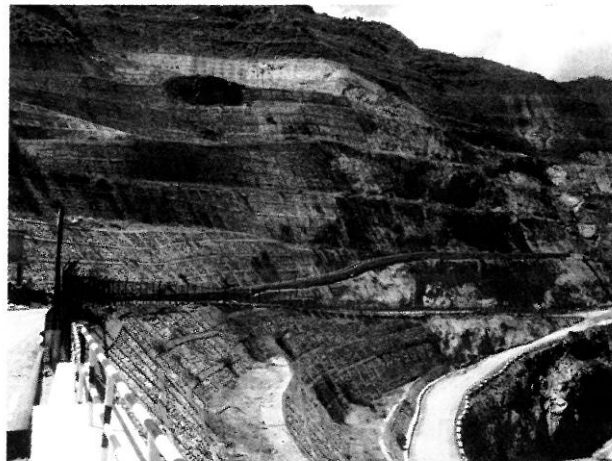
Plate 8 A View of the Treated Slopes at Koteshwar Dam Site
